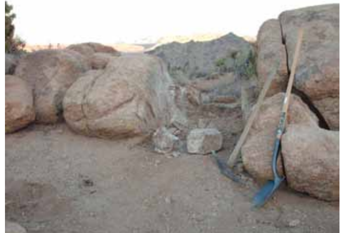
More power! Above left, the untouched top of a ridge shows the general appearance of the Southern California High Desert land. After a good deal of pick and shovel labor, only a small test gap has been opened (above right). When a heavy excavator also couldn’t make progress, holes were drilled out (left) for expanding demolition grout to break the rock up into manageable chunks to be hauled away.
