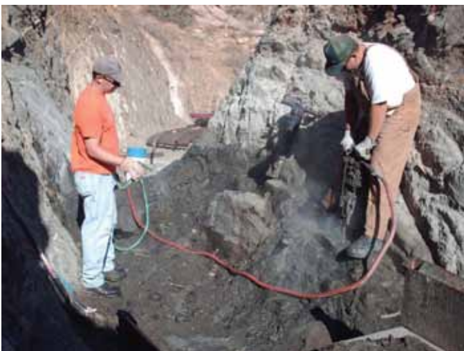
More power! Above left, the untouched top of a ridge shows the general appearance of the Southern California High Desert land. After a good deal of pick and shovel labor, only a small test gap has been opened (above right). When a heavy excavator also couldn’t make progress, holes were drilled out (left) for expanding demolition grout to break the rock up into manageable chunks to be hauled away.
